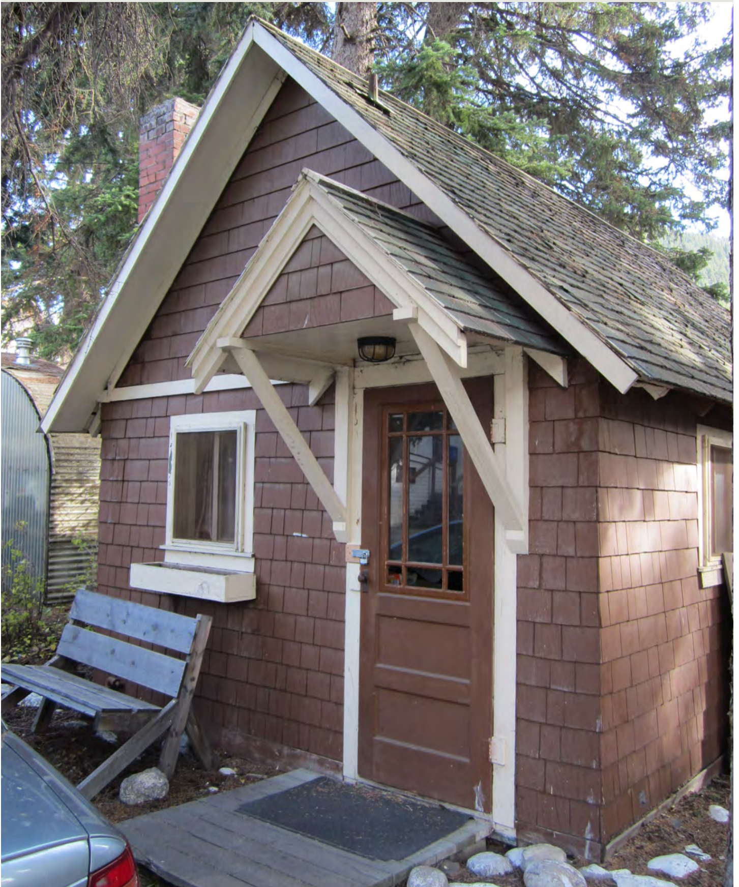
Cabin 1- Main entrance and wooden canopy detailing.
