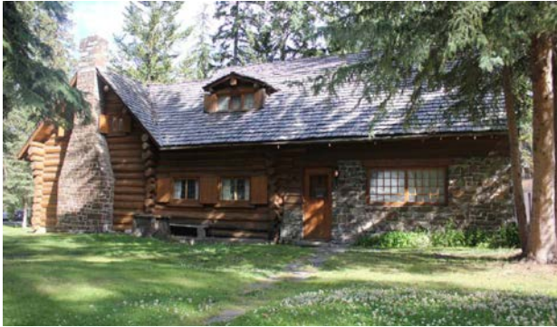
Two storey log cabin
