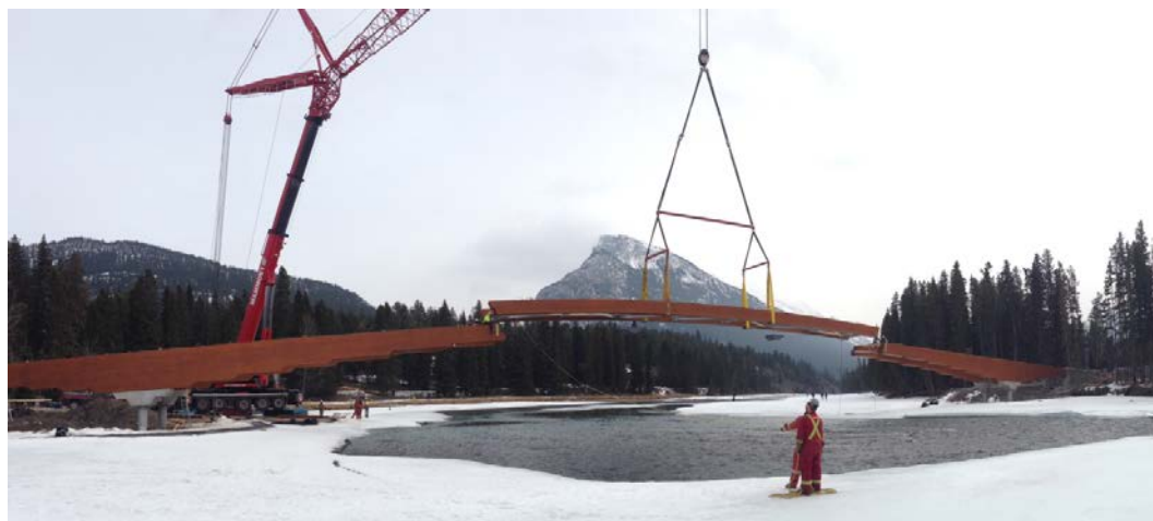
Utility crossing/pedestrian bridge construction in March 2013
