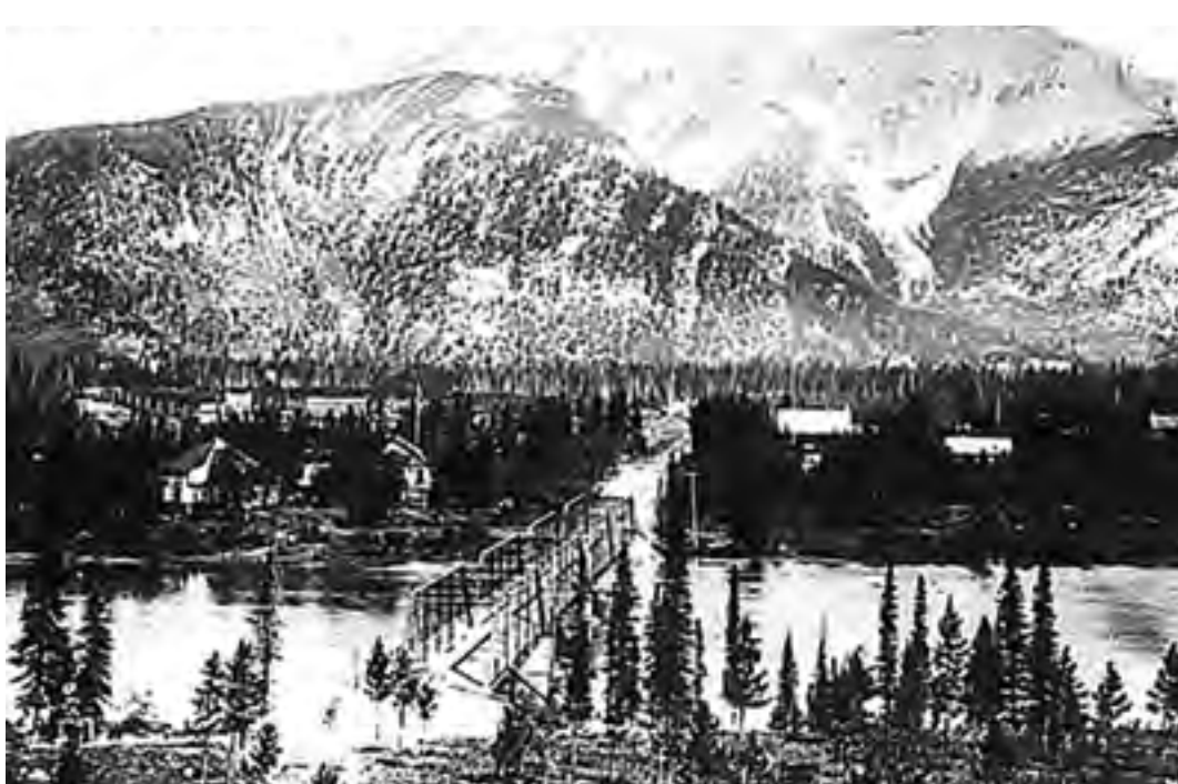
Single-lane iron truss Bow River Bridge.
