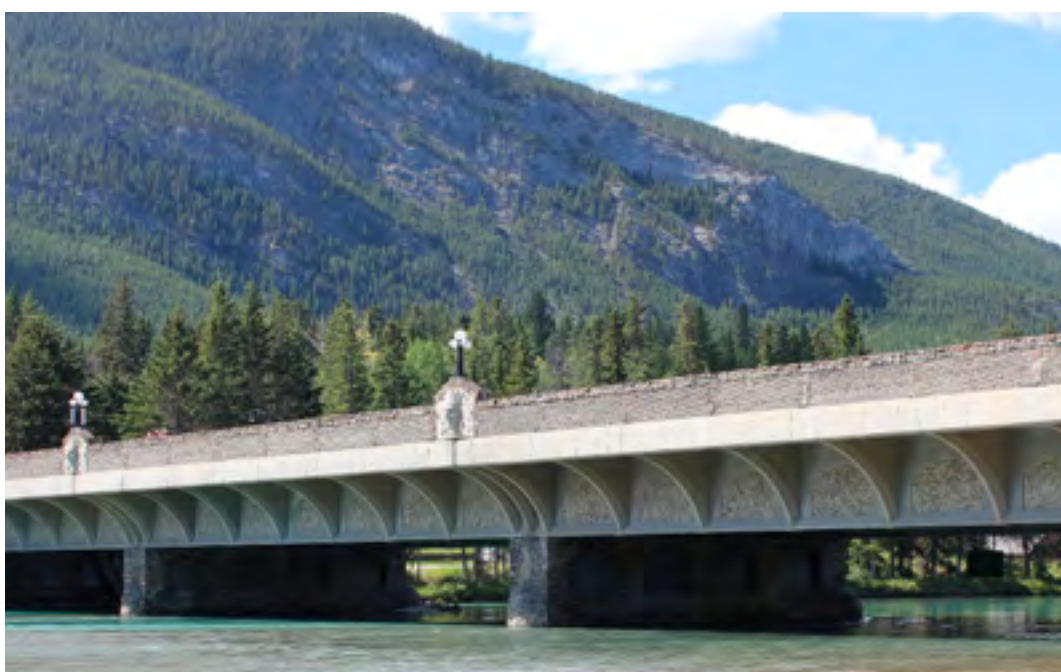
Bow River Bridge present day.
