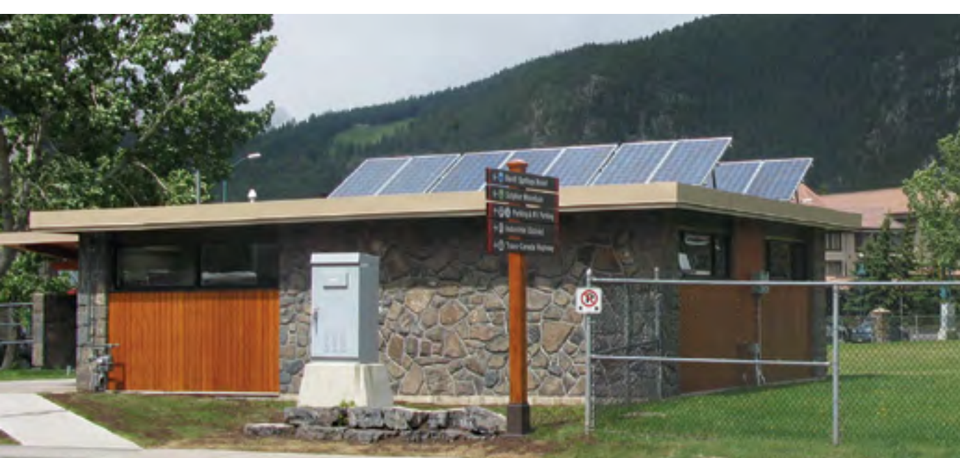
Wolf Street Washroom (3 kW)
